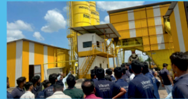
UltraTech Ready Mix Concrete (RMC) Plant, Malanpur
